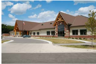
Waunakee Village Center 333 South Madison Street
